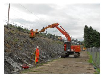
The soil nails were installed with a combination of Klemm KR 904 tracked geotechnical drilling rig and long reach excavator with soil nailing feed beam.
